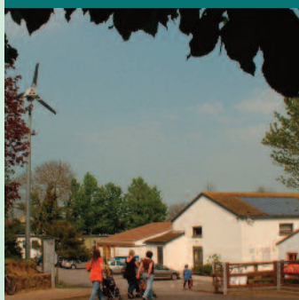
wind turbine and photovoltaic panels
