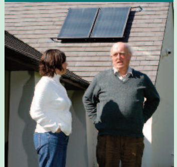
Solar Hot Water panels
