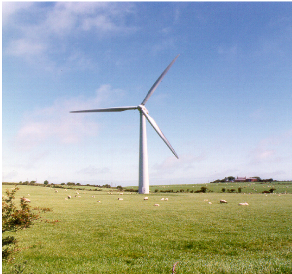
FIGURE 2: A SINGLE LARGER TURBINE
