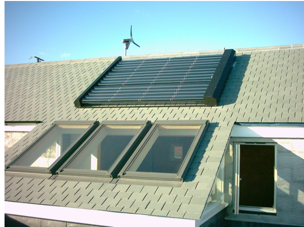
FIGURE 1: INSTALLATION OF EVACUATED TUBES (SOURCE – SOLAR FLAIR)
